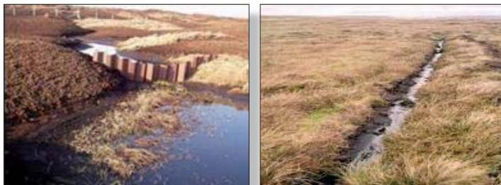
Gully block in erosion channel / Moorland drainage grip
